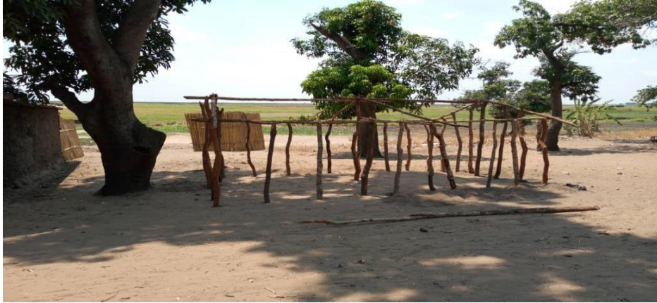
This is a house in making – Young man aged 23 years old was building “his house” on the day of the visitation. This picture (sticks) shows the structure – wall and roof
