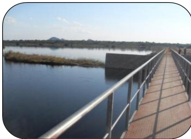
Picture: 13. The foot bridge on the dam can only be used by pedestrians and cyclists
