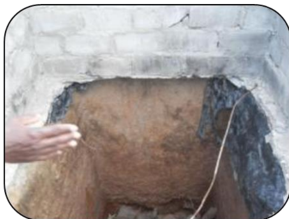
Picture: 11 and 12 One of the seven collapsed VIP latrines
