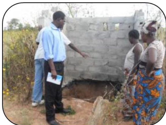
Picture: 11 and 12 One of the seven collapsed VIP latrines
