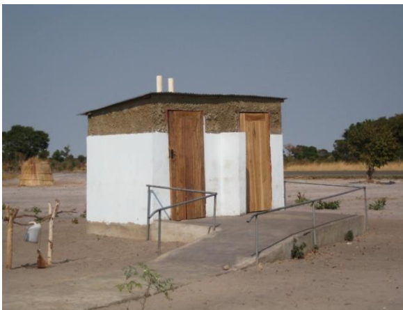
Toilets with slant floors for easy accessibility
