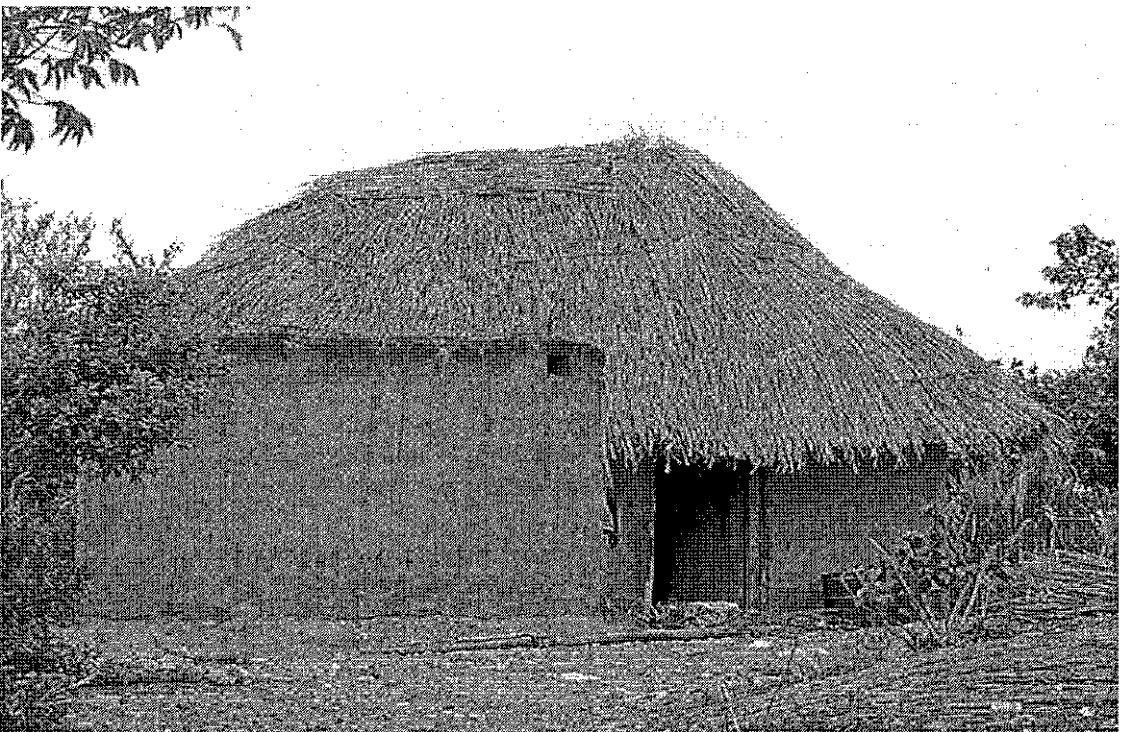
Figure 4: Low cost housing / Traditional housing - Thatched roof, both walls and floor made of mud – Chongwe District
