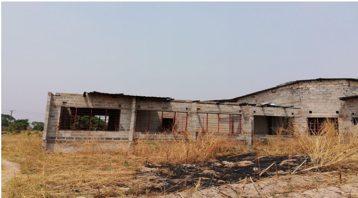
Side view of the police station.
